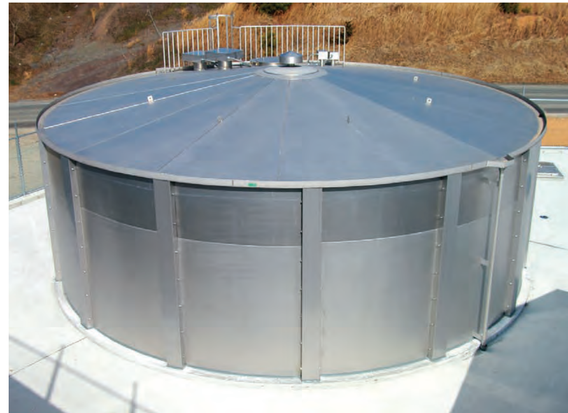
Water supply plant
