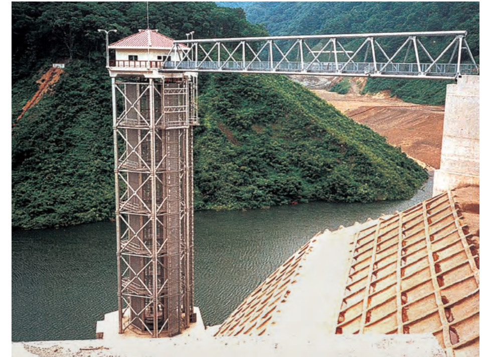
Dam's head gate tower
